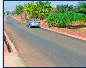
1.15KM STRETCH OF ROAD WITH DUAL DRAINAGE AT ABUDE STREET, AGBOR
